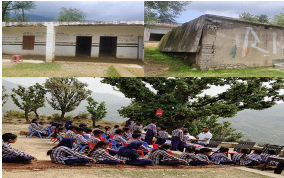
Fig. 1. Students are attending class outdoors due to the collapsed school building.
